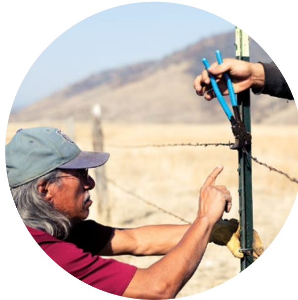
Lands crews replacing fence after fire season.
