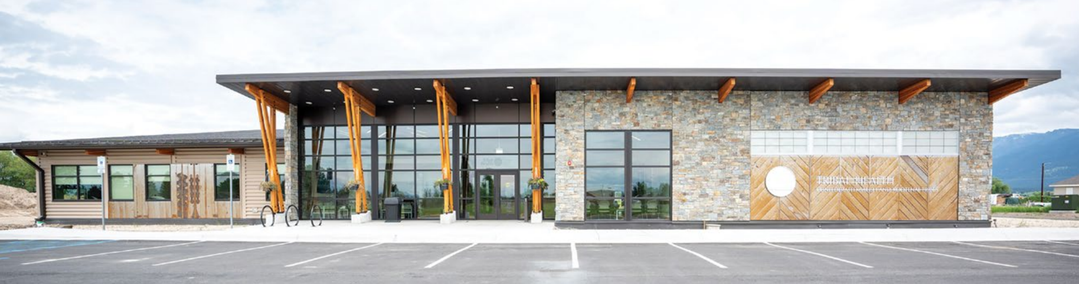
Tribal Health's newest facility, the Ronan Health Center.
