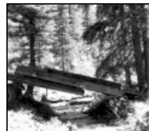
Figure 2-71. A portable railroad flatcar provides access across streams less than 10 feet wide with minimal disturbance to the stream banks or bed. This type of practice is consistent with Best Management Practices.
